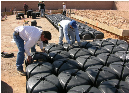
Figur 10a. Cupolex® former placeras ut under bottenplattan.
